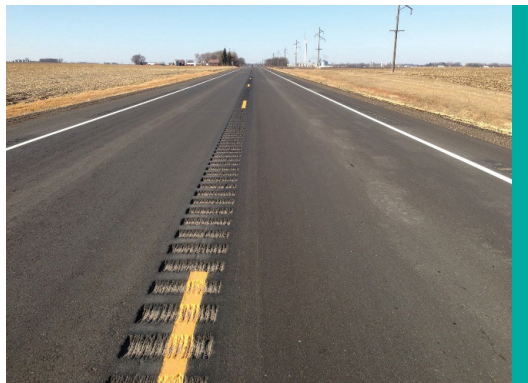
Figure 15. Sample of Installed Milled CLRS (Image: Neal Hawkins)
