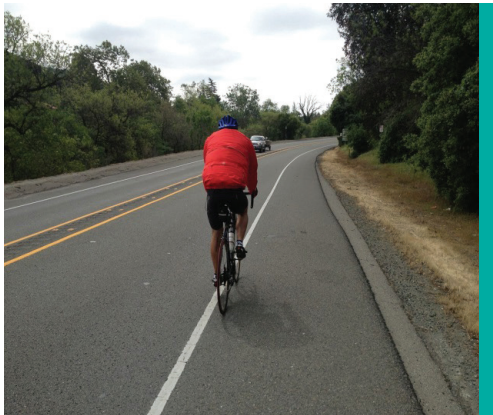
Figure 29. Sample of Wider Shoulder (Image: Caltrans)
