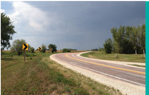
Figure 3. Sample of Installed Chevron (Image: Neal Hawkins)
