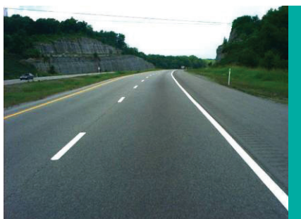
Figure 11. Sample of Installed Edge-Line Pavement Markings (Carlson et al. 2010)
