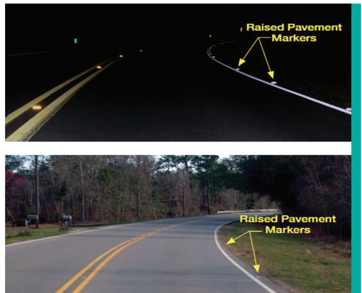
Figure 10. Example of 20-foot RPM Spacing for a Curve During Daytime/Nighttime (FHWA 2013b)
