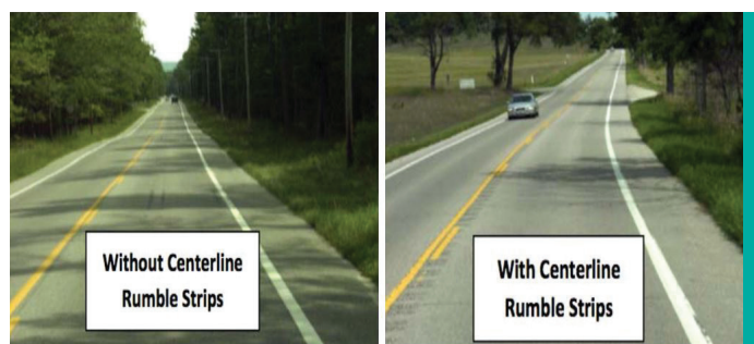
Figure 16. Before (left) and after (right) Pictures of the CLRS Installation (Datta et al. 2012)
