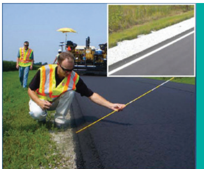
Figure 12. The Safety Edge SM (Image: FHWA)
