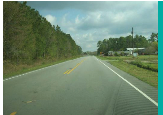
Figure 30. Site 1: Driving North on U.S. 258 (NCDOT 2014)
